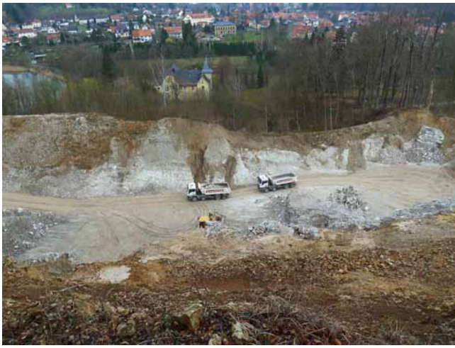
Figure 5. Gypsum quarry destroying the Zechstein landscape south of Walkenried. Photo: Reiner Cornelius.
